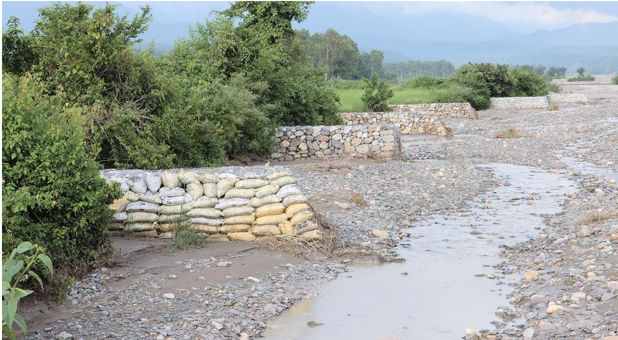
Spurs for controlling flow of torrents
