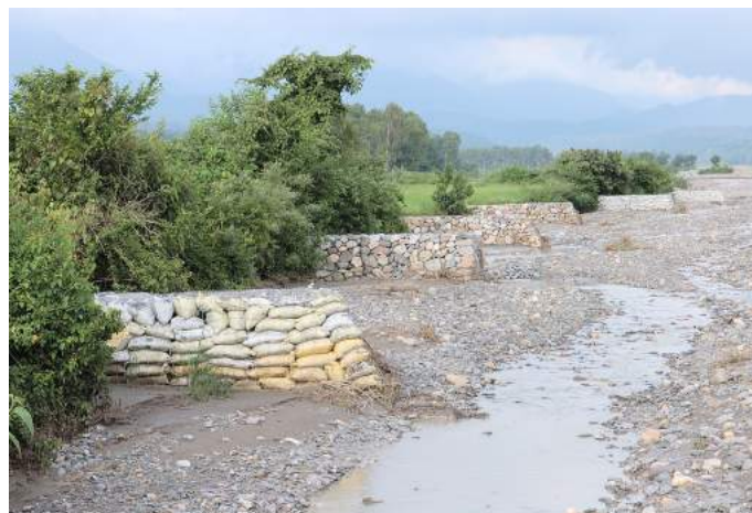
Spurs for controlling flow of torrents
