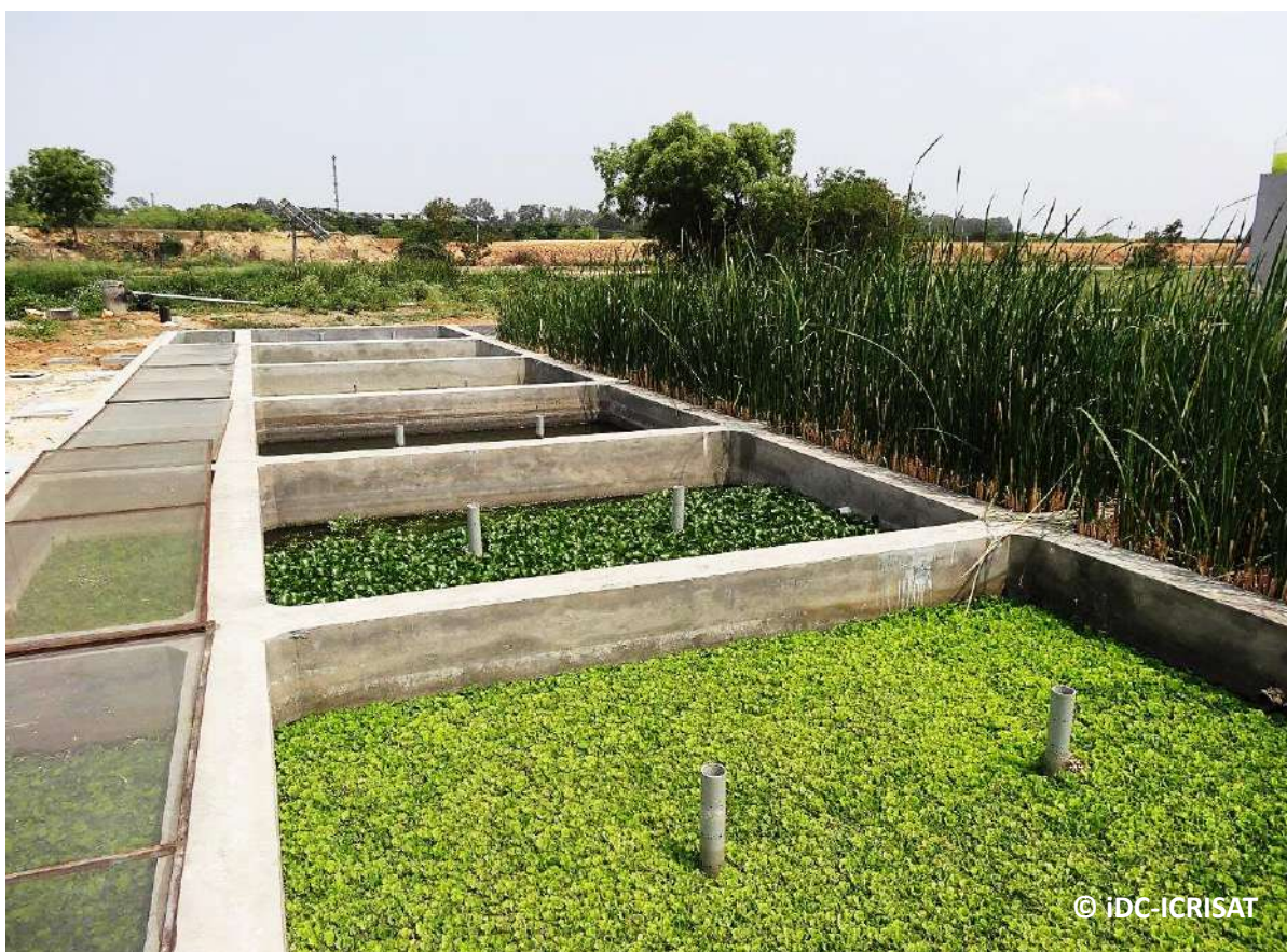
Nature based waste water treatment plant
