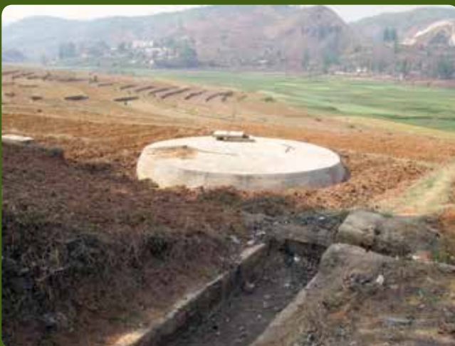
Water tank and irrigation channel in Shuiyan Village
