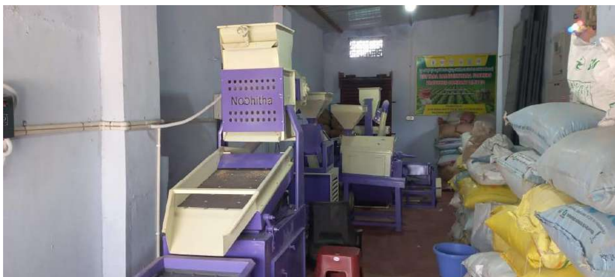
Millet Primary Processing Unit Setup at FPC
